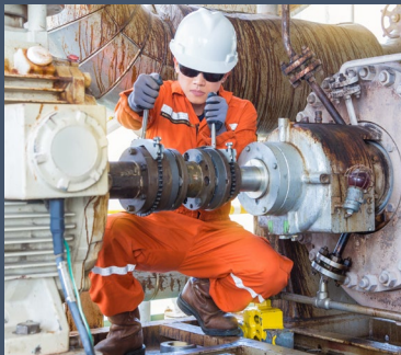
Wrong Coupling Ordered
