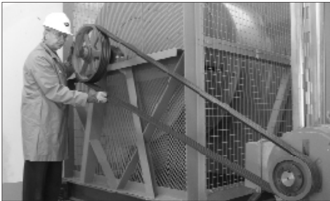
Begin by inspecting the belt
