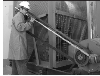
Using a straight edge to check alignment
