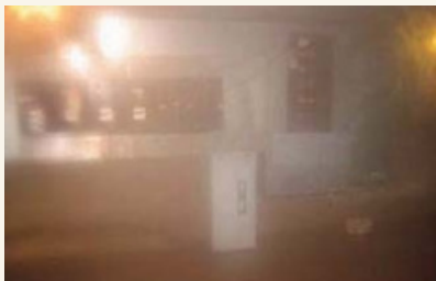
Figure 4 - Major Steam Leak in Basement Area of Garrison Facility (courtesy US Army)
