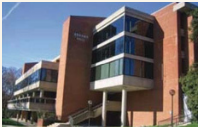
Figure 5 - One of the Barracks Facilities at Walter Reed Army Medical Center (courtesy US Army)
