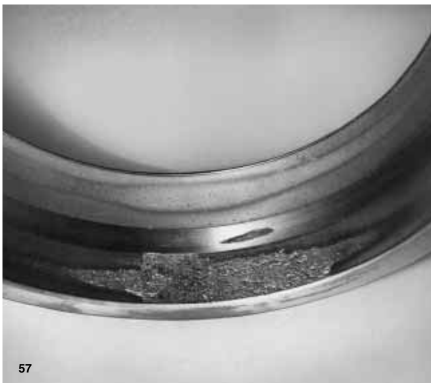
Fig 57 Flaking in the outer ring outer ring of spherical roller bearing that has been mounted in a housing with oval bore
