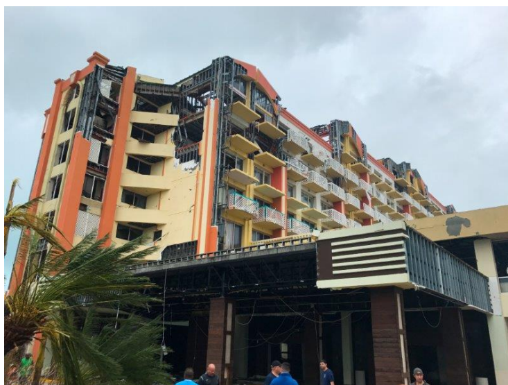
Category 5 Rips through Hotel Building
