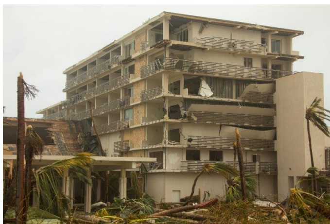
Beware of Falling Debris
