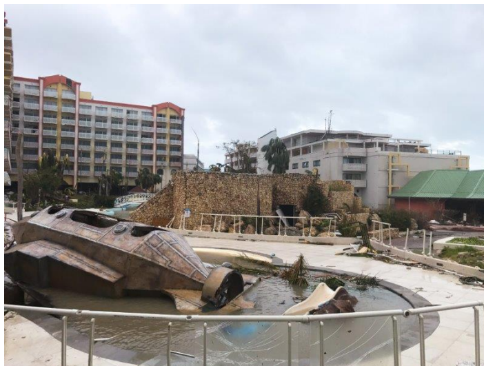
Drain all Pools before the Hurricane
