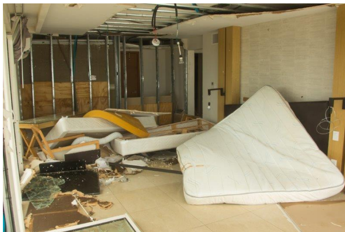
Hotel Room after a Category 5 Hurricane
