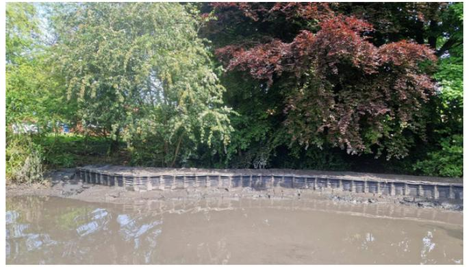
Nicospan fencing installation to form a new embankment for silt deposition.
