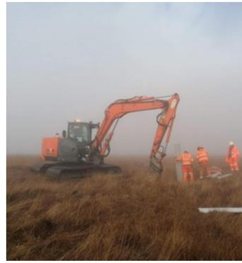
WE HAVE BEEN INSTALLING PEAT AND PLASTIC PILED DAMS USING LOW GROUND PRESSURE EXCAVATORS THAT WILL SERVE AS A NATURAL FLOOD MANAGEMENT TECHNIQUE. THE METHOD ALLOWS FLOOD WATER TO BE HELD UPSTREAM AND RELEASED SLOWLY, LOWERING THE CHANCE OF FLOODING IN DOWNSTREAM AREAS.
