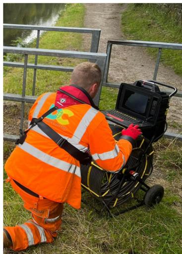
WE HAVE BEEN CARRYING OUT CULVERT CLEARANCE AND MAINTENANCE WORKS ON THE HUDDERSFIELD NARROW CANAL. THE JOB INVOLVED CLEARING THE BUILD UP OF SILT AND DEBRIS FROM THE CULVERTS USING JETTERS. IN ORDER TO ENSURE THE JETTERS WERE USED AT THE CORRECT WATER PRESSURE WE USED CCTV EQUIPMENT TO MONITOR THE EFFECTS OF THE JETTING.
