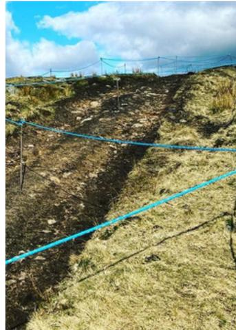
ONE OF OUR TEAMS HAS BEEN AT SWELLANDS RESERVOIR INSTALLING BIRD DETERRENT MEASURES ALONG THE NEW 2KM ACCESS TRACK PRIOR TO CONSTRUCTION WORKS COMMENCING. WE USED GPS SURVEYING EQUIPMENT TO MARK THE NEW ACCESS ROAD AND PASSING PLACES AND THEN INSTALLED 14MM OF BLUE NYLON ROPE IN A ZIG ZAG PATTERN RAISED 1M OFF THE GROUND TO HELP DETER NESTING BIRDS.
