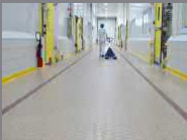
Industrial & Hygienic Floor Application
