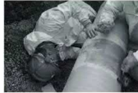
Pipeline Repairing and Rehabilitation
