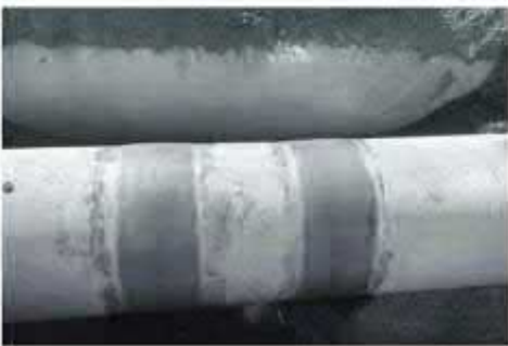
GRP/FRP Lamination[Butt-Wrap]
