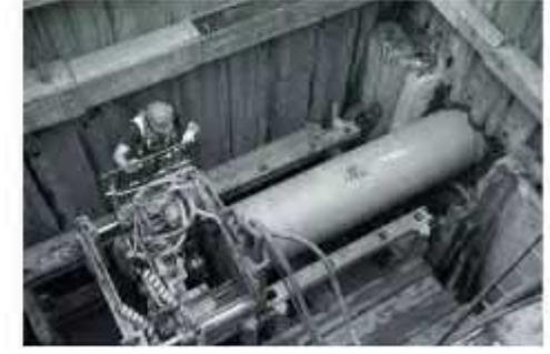
Jacking Pipe / Slip-Lining
