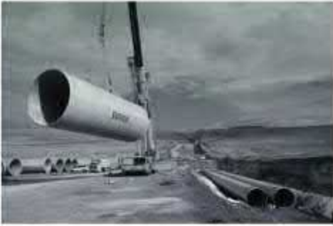
GRP/FRP Pipe Installation
