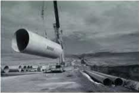
GRP/FRP Pipe Installation
