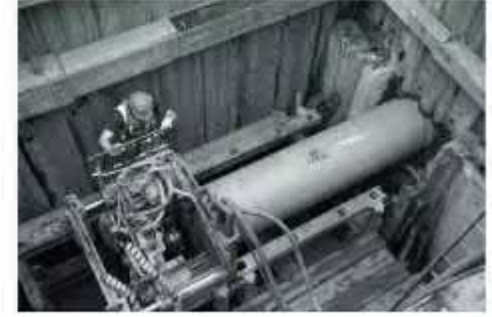
Jacking Pipe / Slip-Lining
