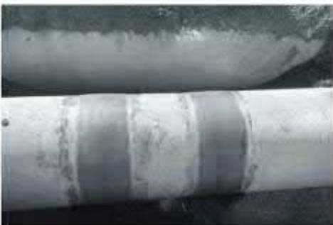
GRP/FRP Lamination[Butt-Wrap]
