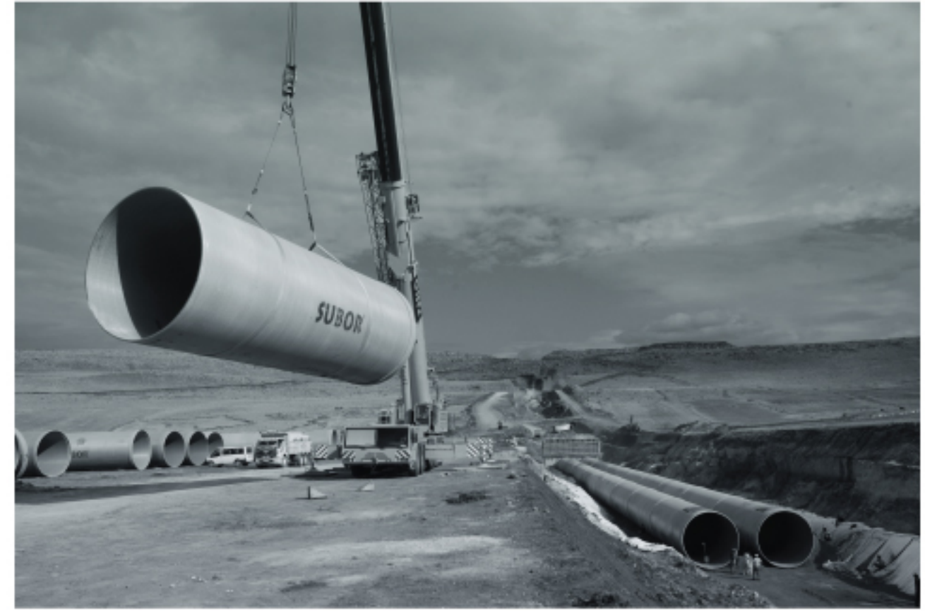
GRP/FRP Pipe Installation
