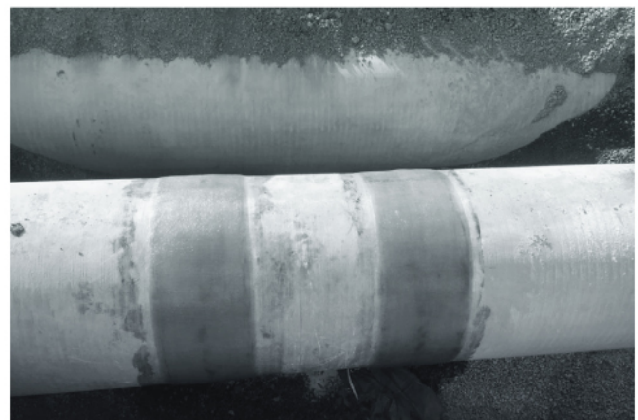
GRP/FRP Lamination(Butt-Wrap)
