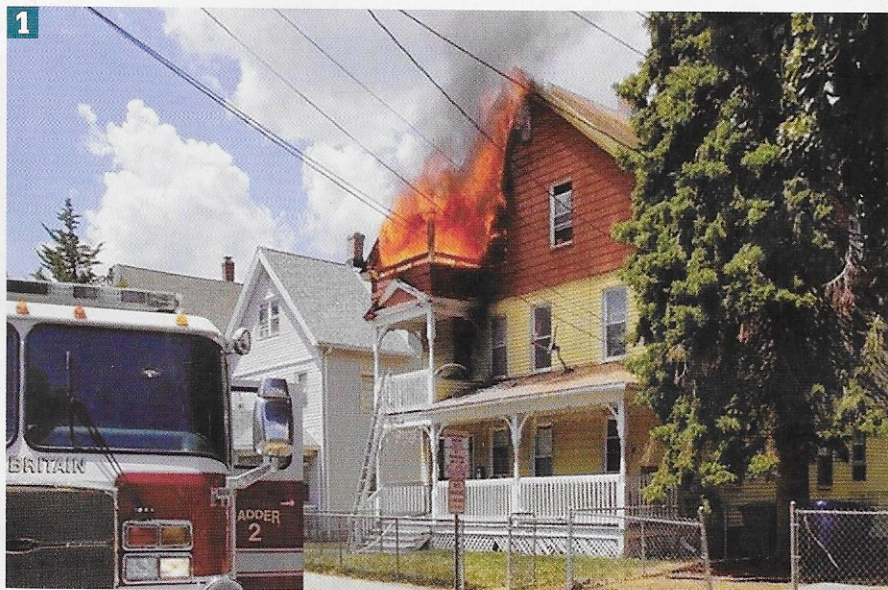
(1) Fire is autoexposing from the front porch and is spreading into the top floor, along the gable, and into the structural void spaces. (Photo by Michael Carena Jr.) (2) The rear porch is well-involved, and fire has extended into the top floor and the structural void spaces. (Photo by Jonathan Turano.)
