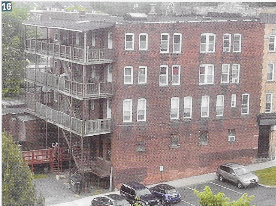
(15) Prompt (coordinated) vertical ventilation was conducted to help confine the fire extension in the attic and limit its horizontal spread. (Photo by Michael Carenza Jr.) (16) The scuttle hatch over the open rear porch and the skylight over the center stairway are visible on the roof of the mixed occupancy—residential (boarding house) over commercial (bar). (Photo by Regina Papa.)
