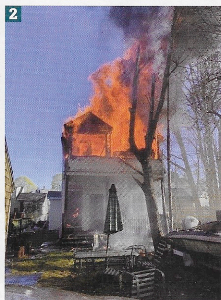
(1) Fire is autoexposing from the front porch and is spreading into the top floor, along the gable, and into the structural void spaces. (Photo by Michael Carena Jr.) (2) The rear porch is well-involved, and fire has extended into the top floor and the structural void spaces. (Photo by Jonathan Turano.)
