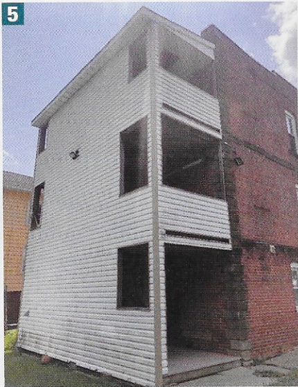
(5) A semi-enclosed rear porch with openings on either end, which would benefit from an angled (“flanking”) position of the handline. (Photos 5–6 by Regina Papa.)
