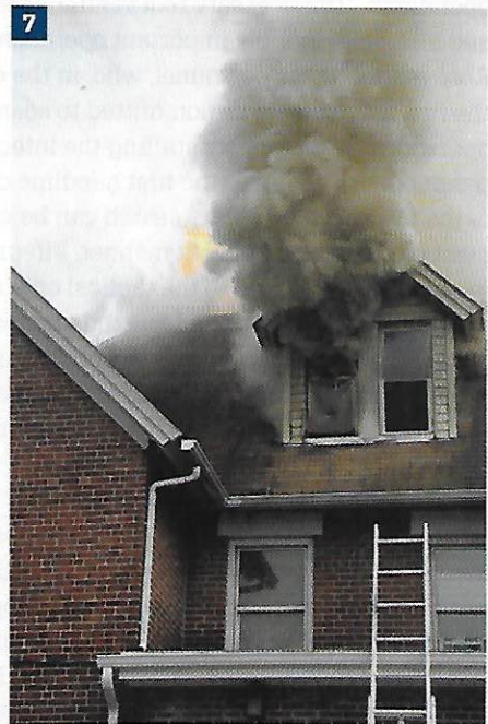
(7) Dormer windows can provide substantial ventilation openings for finished attic spaces. (Photo by Patrick Dooley.)
