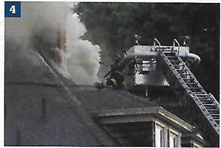
(4) Steep roof pitches and certain construction styles can be problematic for positioning, and they present challenges for access and cutting operations. (Photo by Patrick Dooley.)
