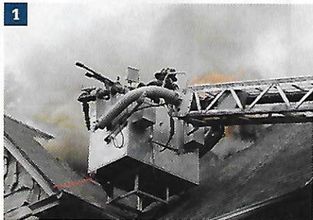
(1) The tower ladder sticks the valley, granting access to multiple sections of the roof, allowing the firefighters to cut both sides from the bucket. (Photo by Patrick Dooley.)
