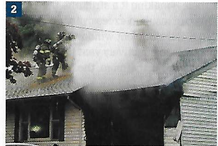
(2) If the vent hole does not have a direct pathway to the fire, it will not be effective in aiding the extinguishment effort. (Photo by Michael Carezza Jr.)
