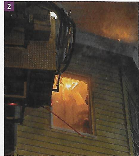
2. The ladder company inside team works to open up the ceilings to expose the fire in the cockloft for the engine company, while the ladder company outside team provides ventilation.
