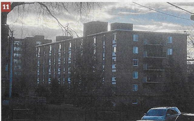
(11) This six-story, center-hallway multiple dwelling of fire-resistive construction has the two bulkheads visible along the roof above the stairways. (Photo by Gina Papa.)
