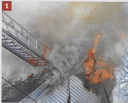
(1) Flames vent from the gable end of a peaked-roof dwelling and smoke is pushing from the eaves and from underneath shingles, indicating an advanced fire involving the structural void spaces. (Photo by Pat Dooley.)
