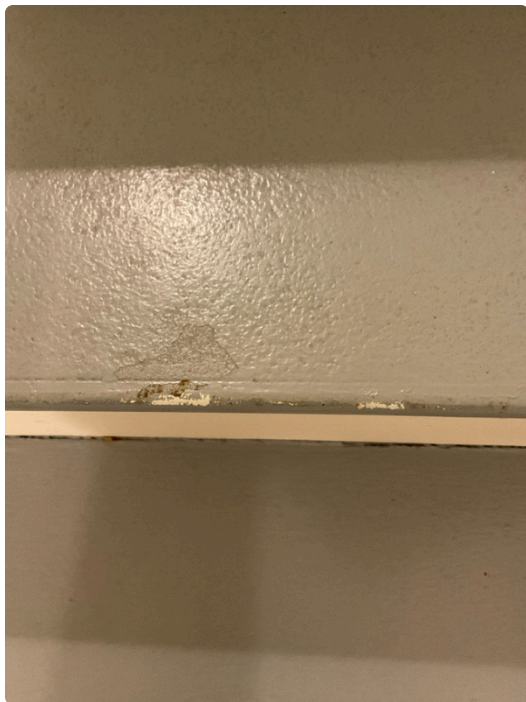
Edge chipping at the south stairs at 2nd floor
