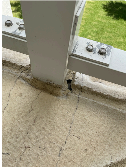
Cavity at the base of the railing post between units 301 and 302
