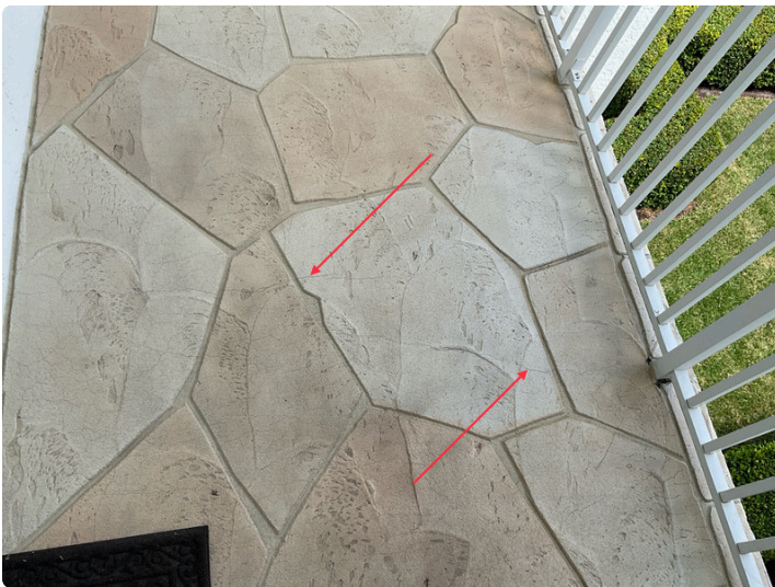
Cracks on walkway at unit 203
