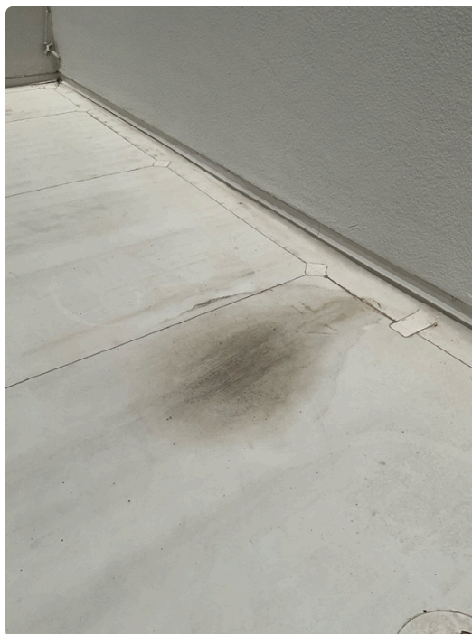
Water stain indicating water pooling at the roof
