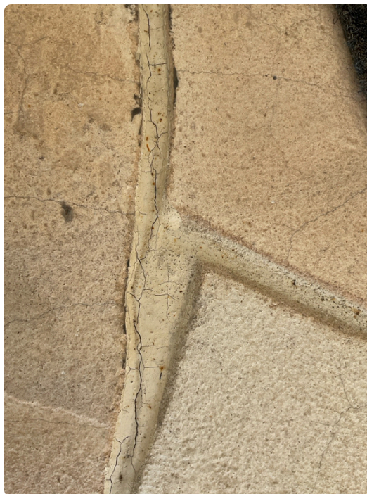
Crack on the sealant
