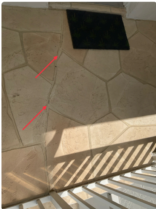
Crack on the sealant by unit 102
