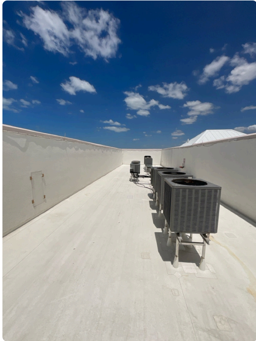
TPO roof surface in good condition
