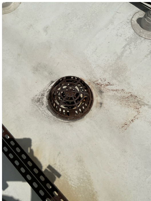
Corrosion on drain screen at the roof
