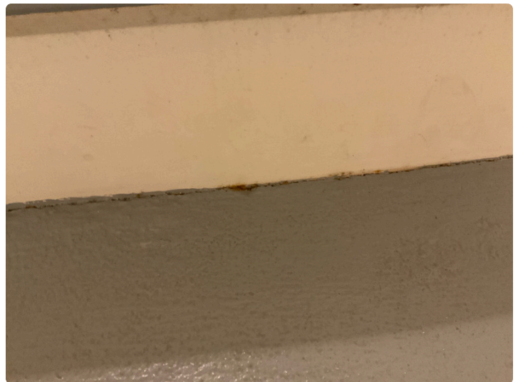
Signs of corrosion at south stairs at 3rd floor
