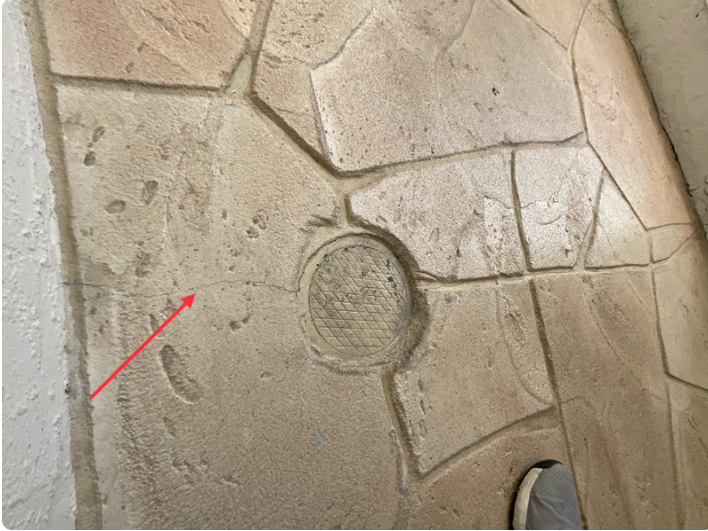
Crack on the walkway at ground floor between storage rooms and south stairwells
