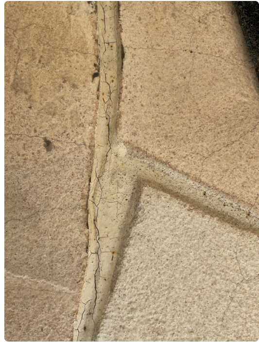
Crack walkway grout by unit 102
