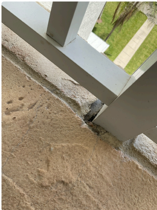
Cavity at the base of the railing post between at unit 402
