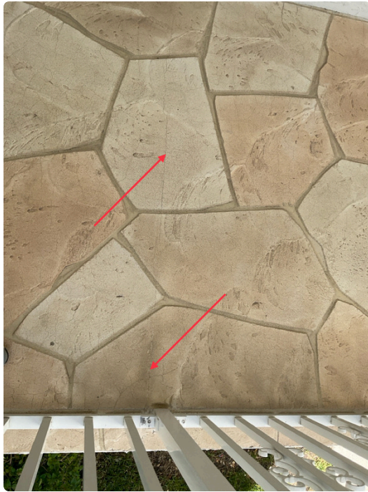
Crack on walkway between units 101 and 102
