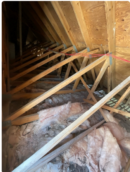
Mansard interior reveals wood structure
