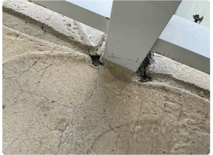
Cavity at the base of the railing post between units 301 and 302
