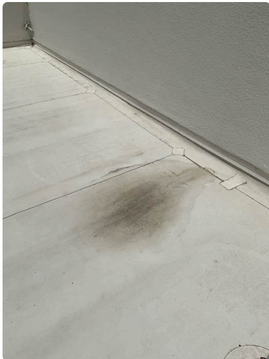
Water stain indicative of water pooling issue
