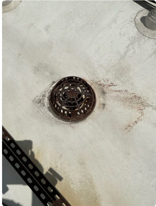
Corrosion on drain screen
