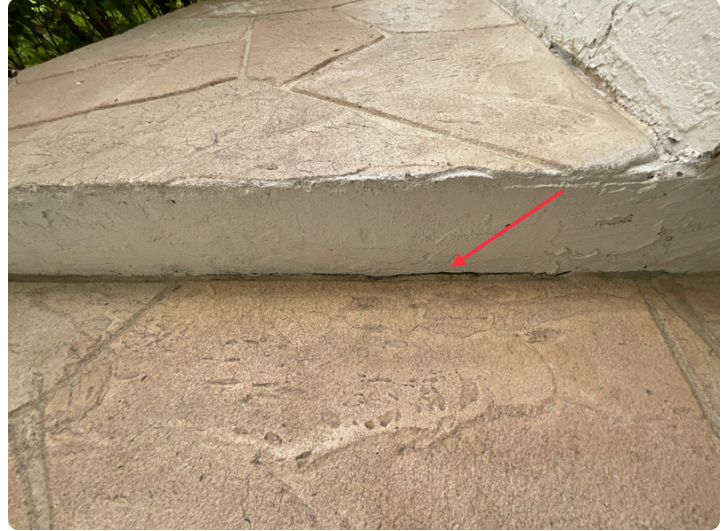
Gap at slab and walkway interface at ground floor, between storage rooms and south stairwells
