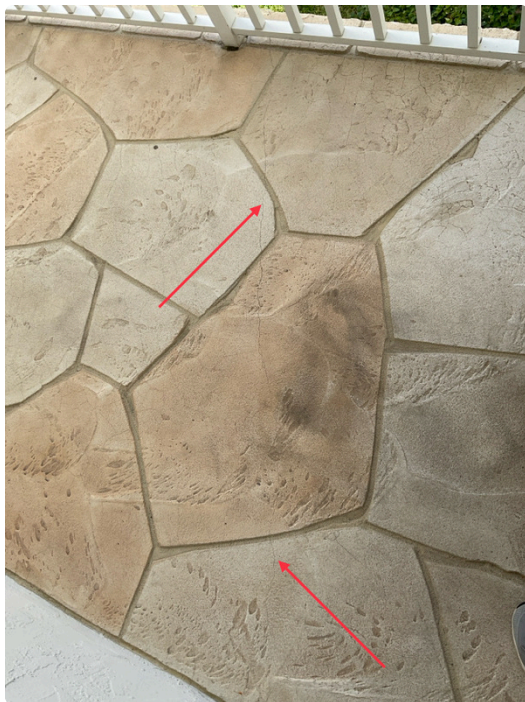
Cracks all over the walkway extending from wall to edge at unit 101
