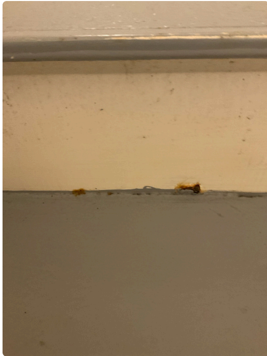
Signs of corrosion at south stairs at 3rd floor
