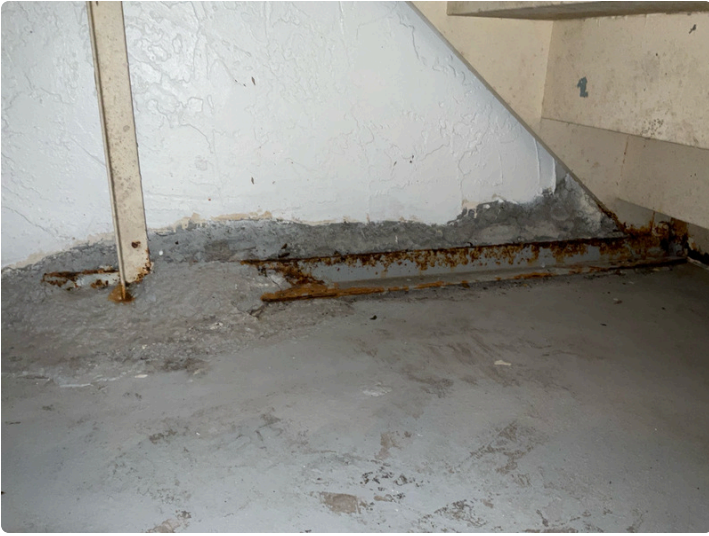
Corrosion on metal constituent of the south stair at ground floor
