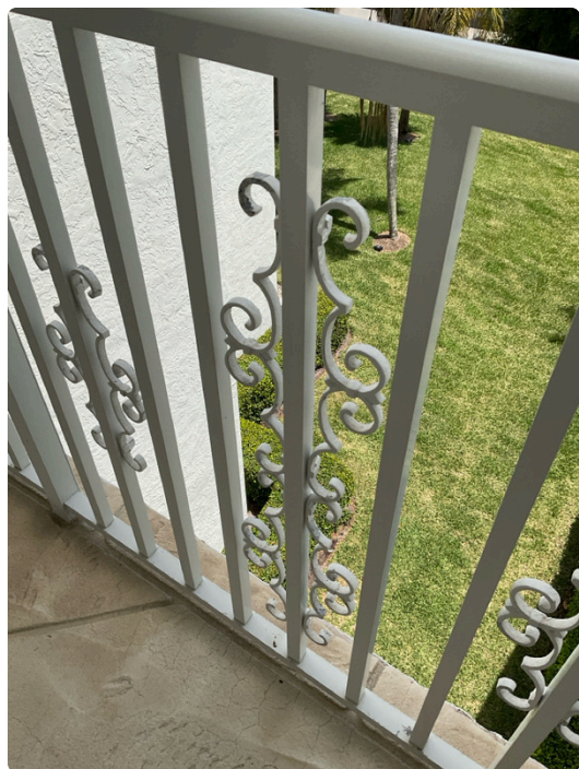
Loose railing decoration at unit 303
