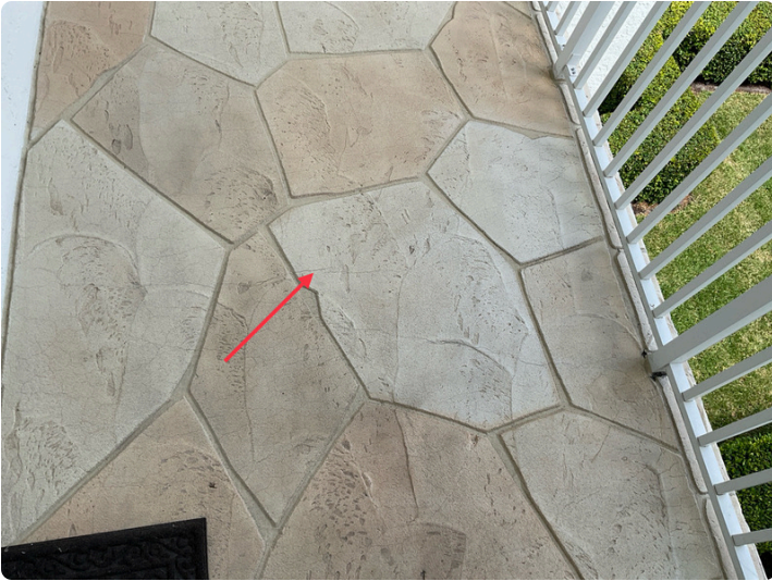
Cracks on walkway by unit 203
