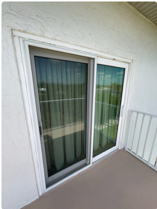
Balcony slider waterproofing in good condition
