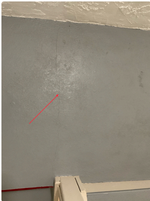
Crack on the landing of north stairs between 3rd and 4th floor
