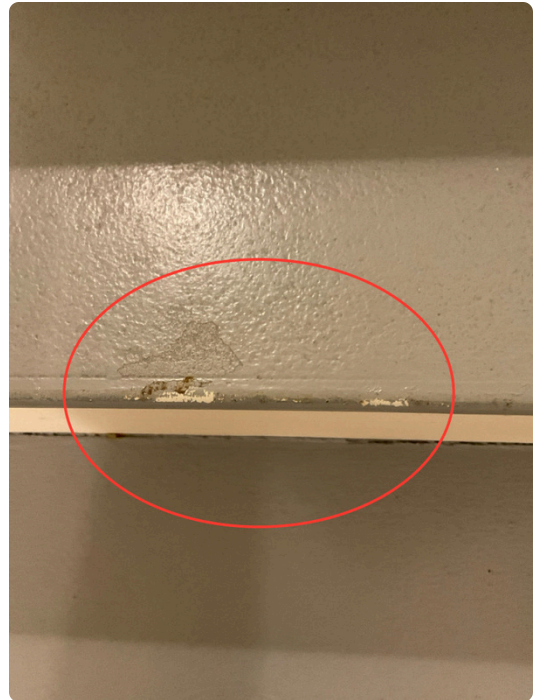
Edge chipping at the south stairs at 2nd floor
