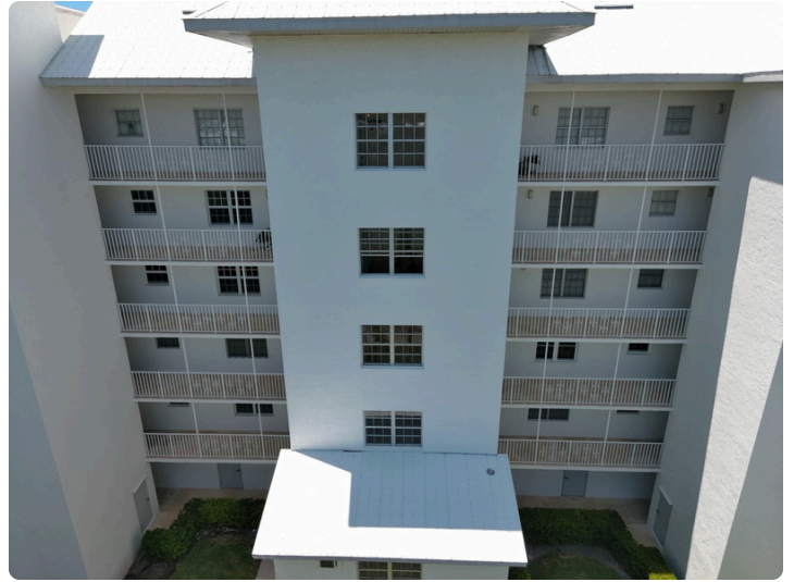
Wall waterproofing in good condition
