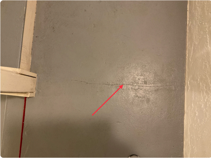
Crack on the landing of south stairs between 3rd and 4th floor
