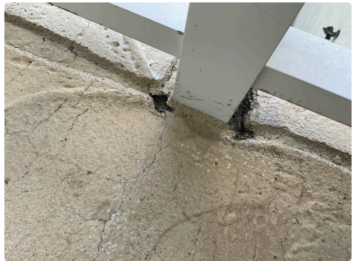
Cavity at the base of the railing post between units 201 and 202
