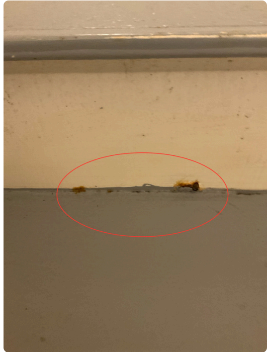
Signs of corrosion at south stairs at 3rd floor
