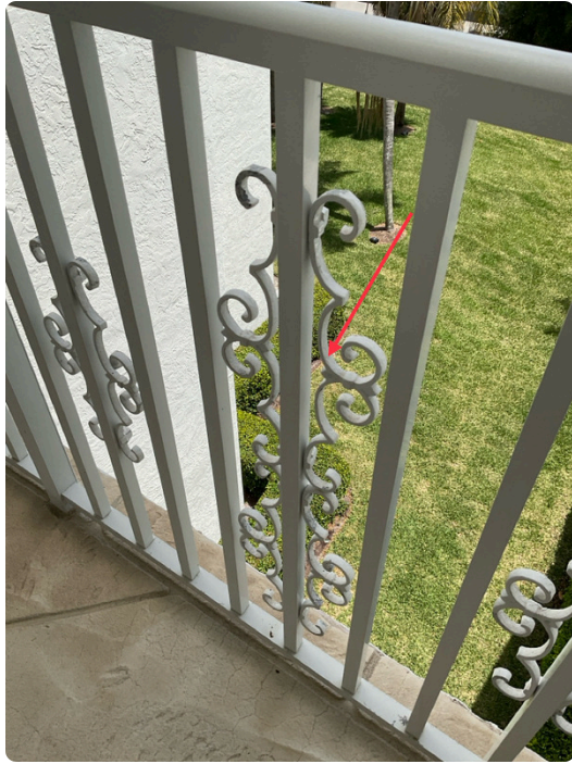
Loosely attached railing decoration infill at unit 303
