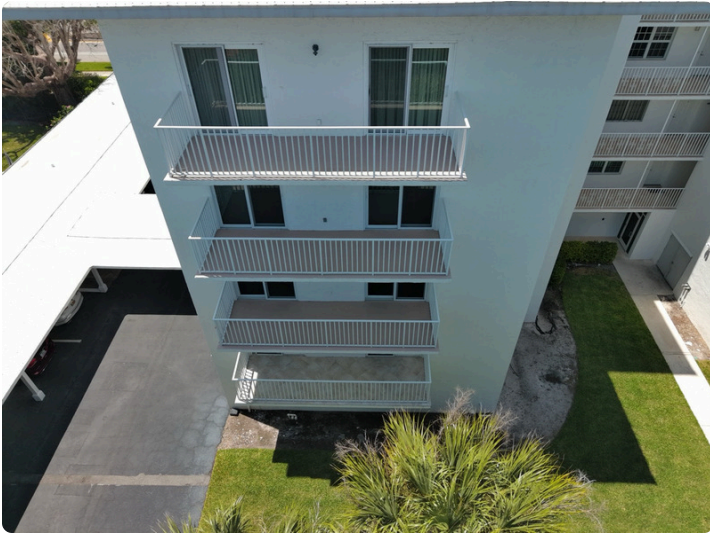
Balcony waterproofing in good condition
