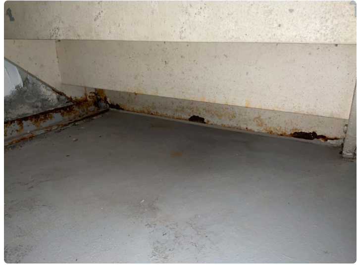
Corrosion on metal constituent underneath the treads of the south stair at ground floor
