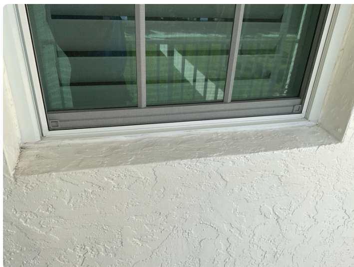
Window sealant in good condition
