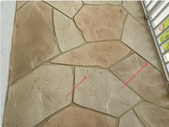
More cracks on the walkway on 3rd floor
