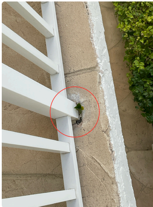
Cavity at the base of the railing post between units 101 and 102
