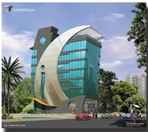
Project Name : Corinthian Location : Khar, Mumbai Area : 75,000 Sq. Ft. Client : DLH (Dev Constructions)
