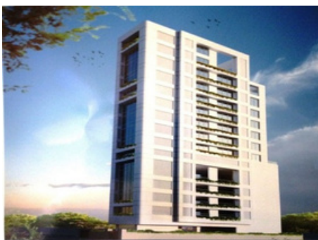
Project Name : Shreeji Homes, Location : Dadar west Area : 75000 Sq ft Client : Shreeji homes
