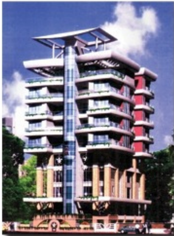
Project Name : Nanak Niwas Location : J.V.P.D Mumbai Area : 22,000 Sq. Ft. Client : DLH (Dev Construction)
