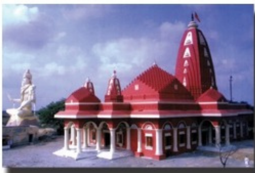
Project Name : Shri. Nageshwar Temple Location : Nageshwar, Gujarat Client : Shri. Gulshan Kumar Charitable Trust
