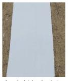
Coating over the fabric should completely hide the joint and fabric.
