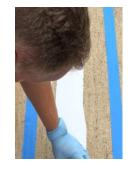
Roll out the **RepTape CT** into the basecoat without elongating the fabric.
