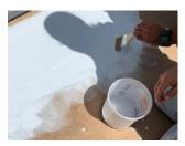
1. Broadcast 16/30 or 12/20 mesh round silica sand at 80 percent of refusal into wet basecoat (confirming sand doesn't sink) at 15lbs-20lbs/100SF (cover the entire area of the deck).
