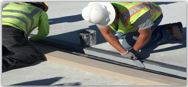
**RepPoxy PA** is a two component, low odor, low viscosity, fast setting, epoxy primer with unique penetrating characteristics. It is designed to enhance the adhesion between substrates, sealants, and topcoats. **RepPoxy PA** seals porous surfaces to prevent pinholes and also performs as a lubricating adhesive for foam and rubber joints. This primer can be used on concrete, steel, plywood and in heavy traffic areas. Use for indoor or outdoor applications.
