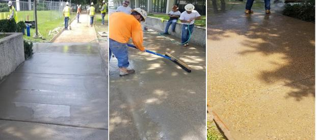
PrepEtch<sup>TM</sup> gave an excellent, evenly exposed etch, on the freshly poured colored aggregate finish at the new NASA Historical Green Space at Space Center Houston! (Mockup surfaces were pretested to determine the square feet per gallon ratio required to achieve the depth of etch desired.)
