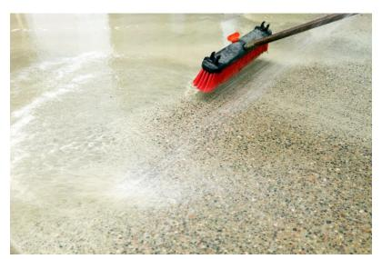
PrepEtch<sup>TM</sup> has been used as a concrete retarder for exposed aggregate!
