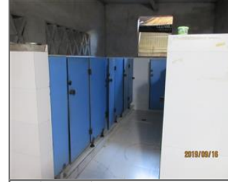
Photo of the sanitary facilities Toilet.JPG
