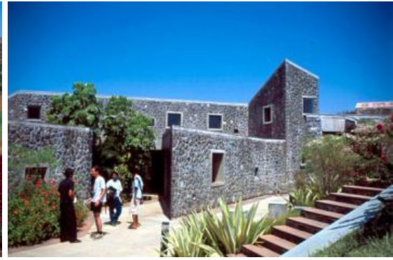
The administrative building reflects the Architectural language of the campus
