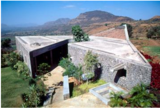
The library twists a light atrium into the Center of the structure
