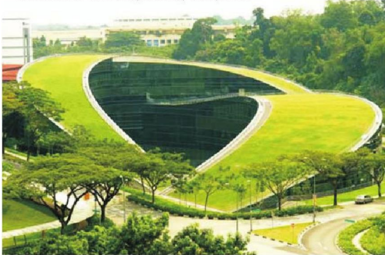
Aerial view of the school
