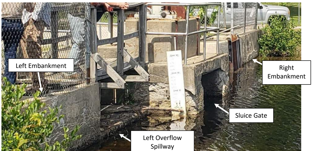
Photo No. 4 – Close up view from discontinued intake structure, looking right. Note concrete loss on the gate structure. Note the difference in the height of the spillway crest above the headwater of the right overflow spillway (pictured in the previous photo) and the left overflow spillway (pictured here).
