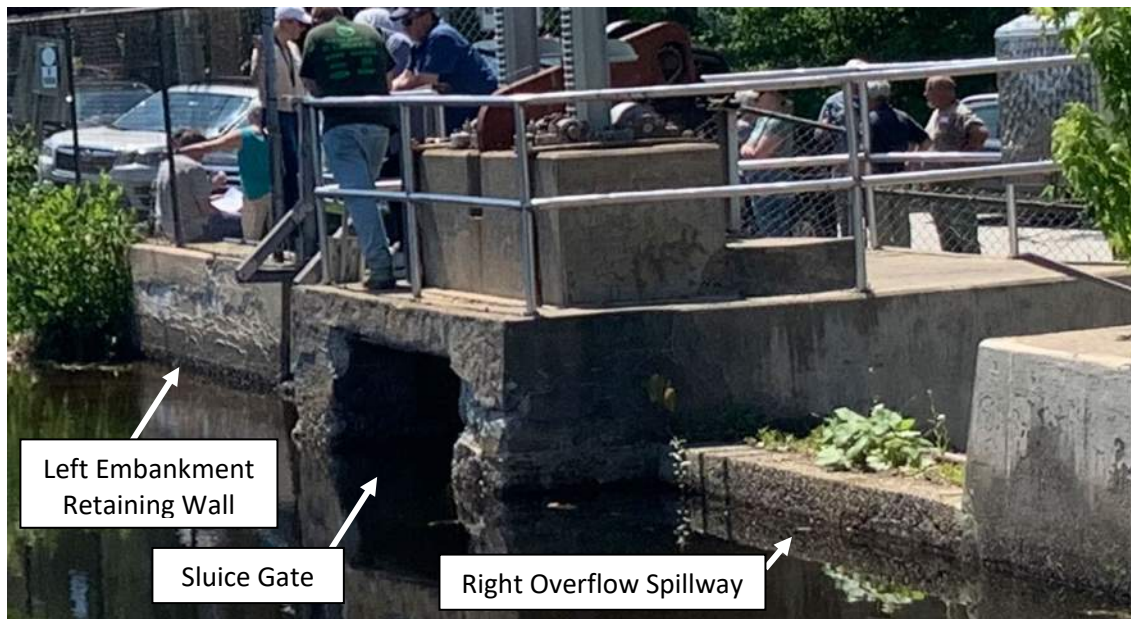
Photo No. 3 – Close up view from right upstream shore, looking left/downstream. Note concrete loss on gate structure and left embankment upstream retaining wall. Note the difference in the height of the spillway crest above the headwater of the right overflow spillway (pictured here) and the left overflow spillway (pictured in the following photo).
