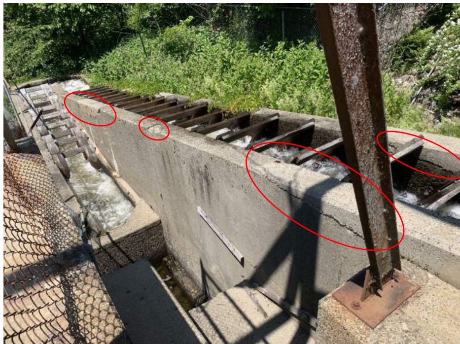
Photo No. 11 – View of fishway from operator platform. Evidence of prior concrete repairs visible. Some concrete spalling.
