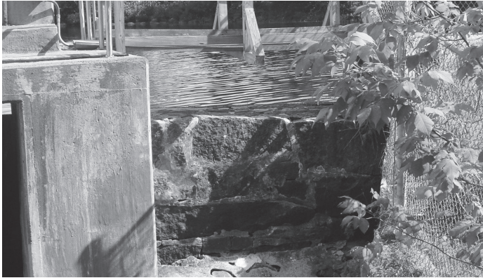
West overflow spillway, August (before the storm)
