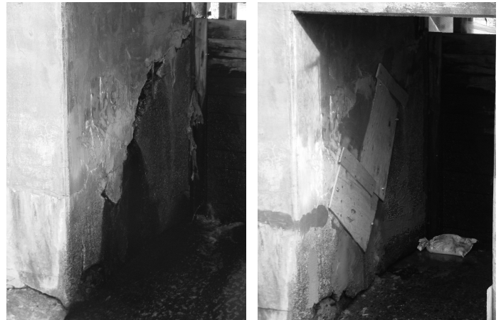
East pier on September 26 (left) and on October 26 (plywood forms to be removed after concrete has set up).
