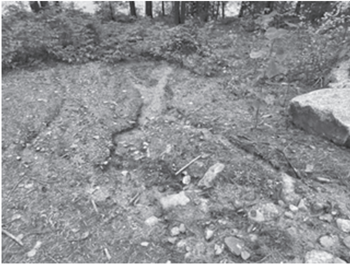
Runoff from our property ...
