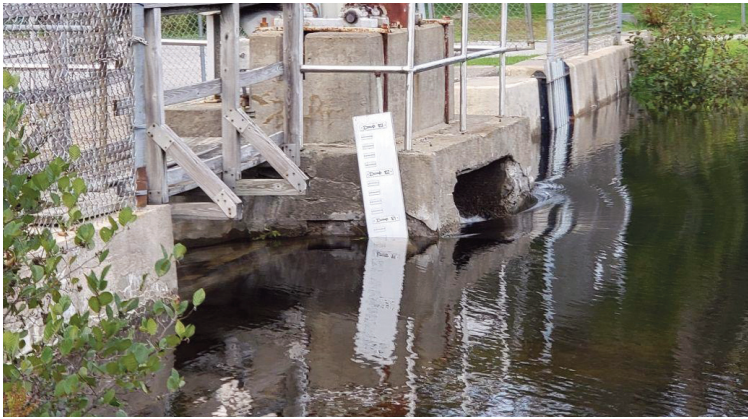
Back side of dam with staff gauge
