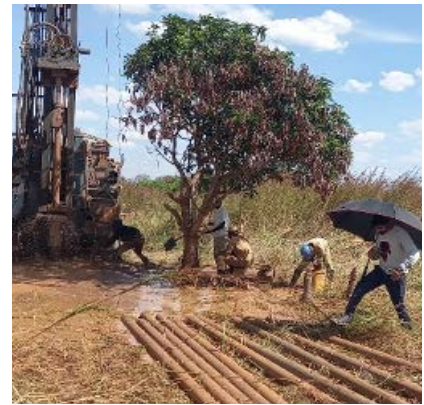
A drilling team builds a borehole.
