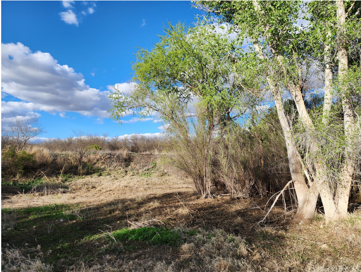
Figure 16 - Borrow pit needs to be regraded to function properly as a wetland, as well as improve safety for users walking in the area.
