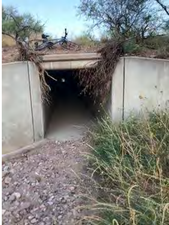
Box culvert under I-19 much larger than the 3 CMPs at Anza Trail ( outlet to river ). (Photo by Rich Kiker)
