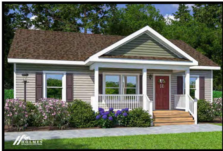
Elevation Shown with Optional and On-Site Builder Supplied Items. Consult Your Builder for Pricing.
