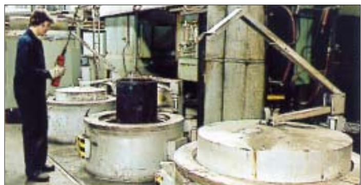
Convection type tempering furnace
