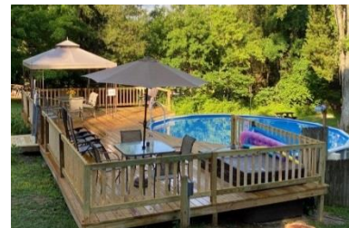
New pool deck, built 2020
