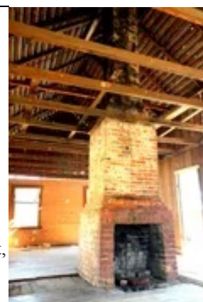
The interior chimney. The fireplace faces two rooms. (photo by Wanda Carole Wrinkle Ford)
