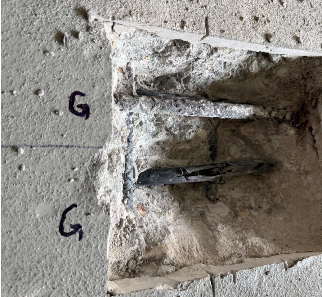
Photo 5: Cut in Tendon Sheathing
