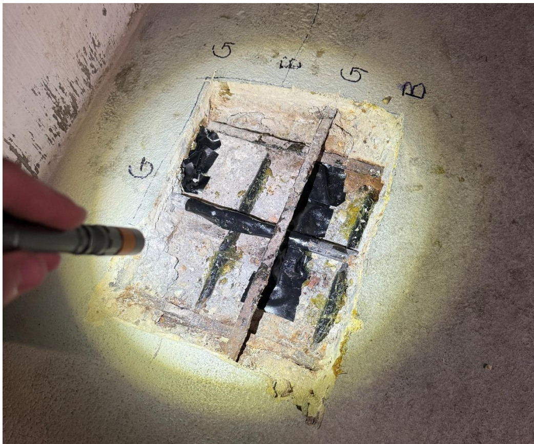
Photo 8: Tendon Protection Where Tendon Could Not be Fully Wrapped
