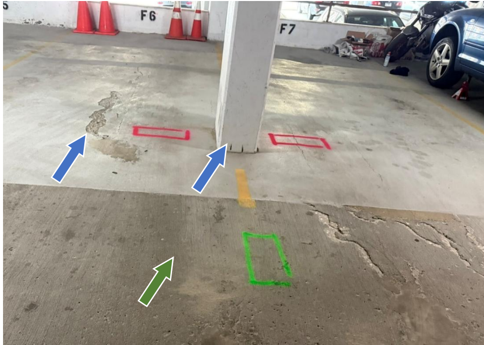
Photo 1: Main Tendon Location Markings – Green Arrow Indicates Temperature Tendon Location Marking
