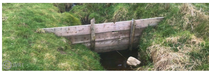
Figure 10 One of the NFM interventions used within the Wyre is leaky barriers. Designed with gaps to slow water flow at peak rainfall events, reducing the likelihood of flash flood events.
