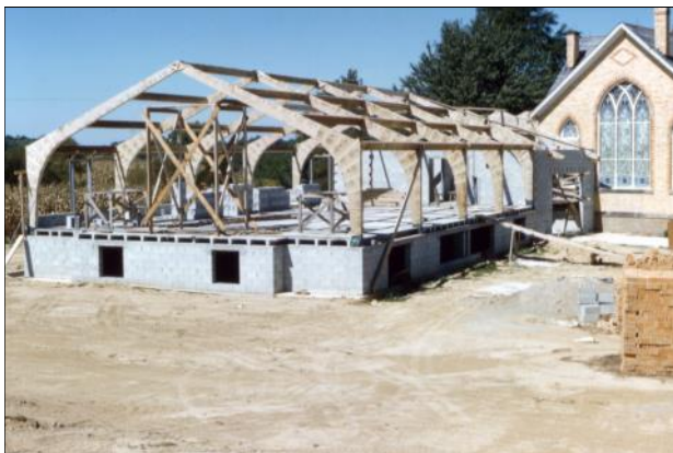
Wooden roof trusses in place.
