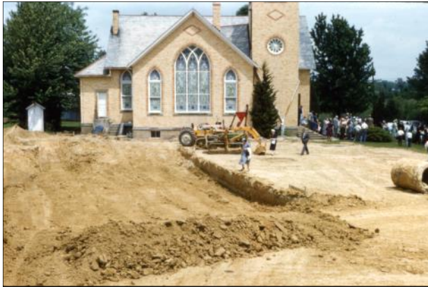
Excavation for the Parish Hall begins.
