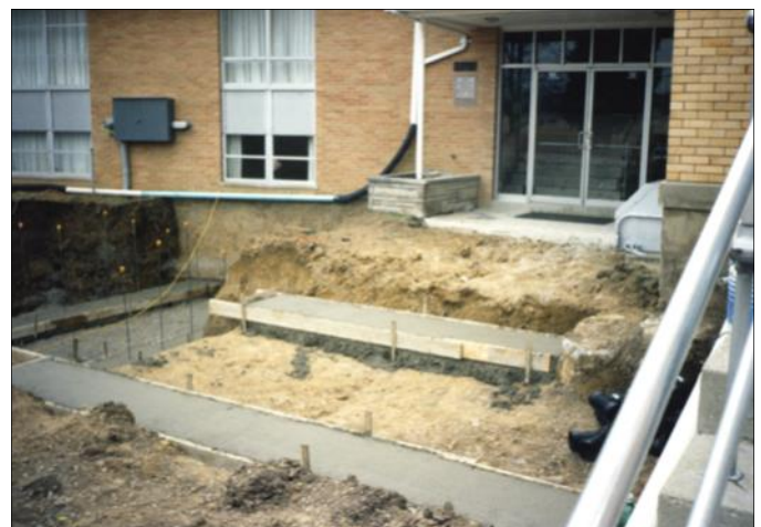
Construction of the Access Improvement Facility.
