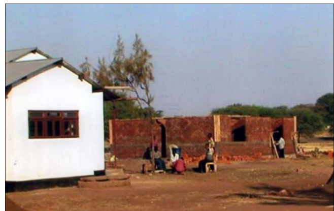
Construction of the Home of Peace Orphanage in Bariadi, Tanzania.
