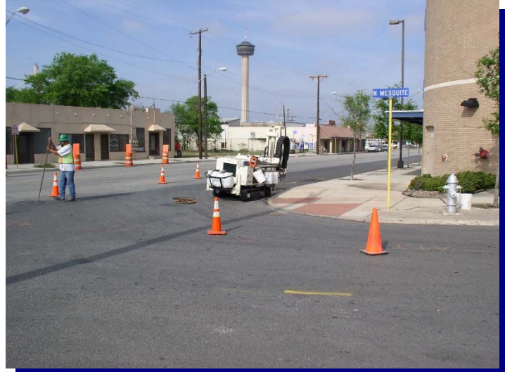
Commerce Street Phase II ESA
