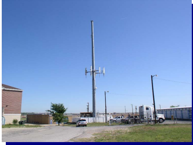
Tower under construction
