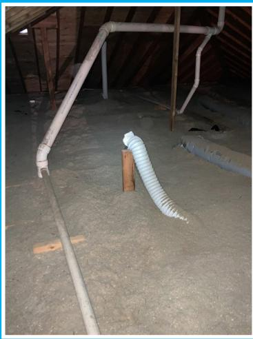
**Prior to 2006, bath exhausts did not have to vent outside. A home inspector will require this to be updated. We can install duct and vent it to the outside of your home per code.**
