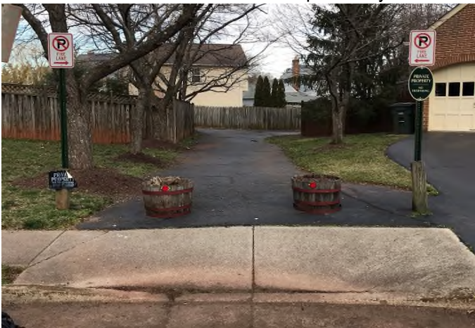
The association is responsible for the fire lane. See our recommendations in the comments section for proper care of asphalt pavements.
