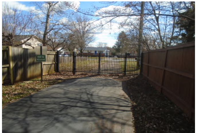
Gates on backside of fire lane will repair and replacement at end of useful life.
