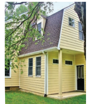
▶ An ATTACHED ADU connects to an existing house, typically through the construction of an addition along the home’s side or rear. Such units can have a separate or shared entrance.
