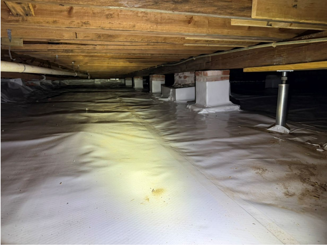
Exhibit A.2: Moisture Damaged Beams and Joists With Temporary Supports Added
