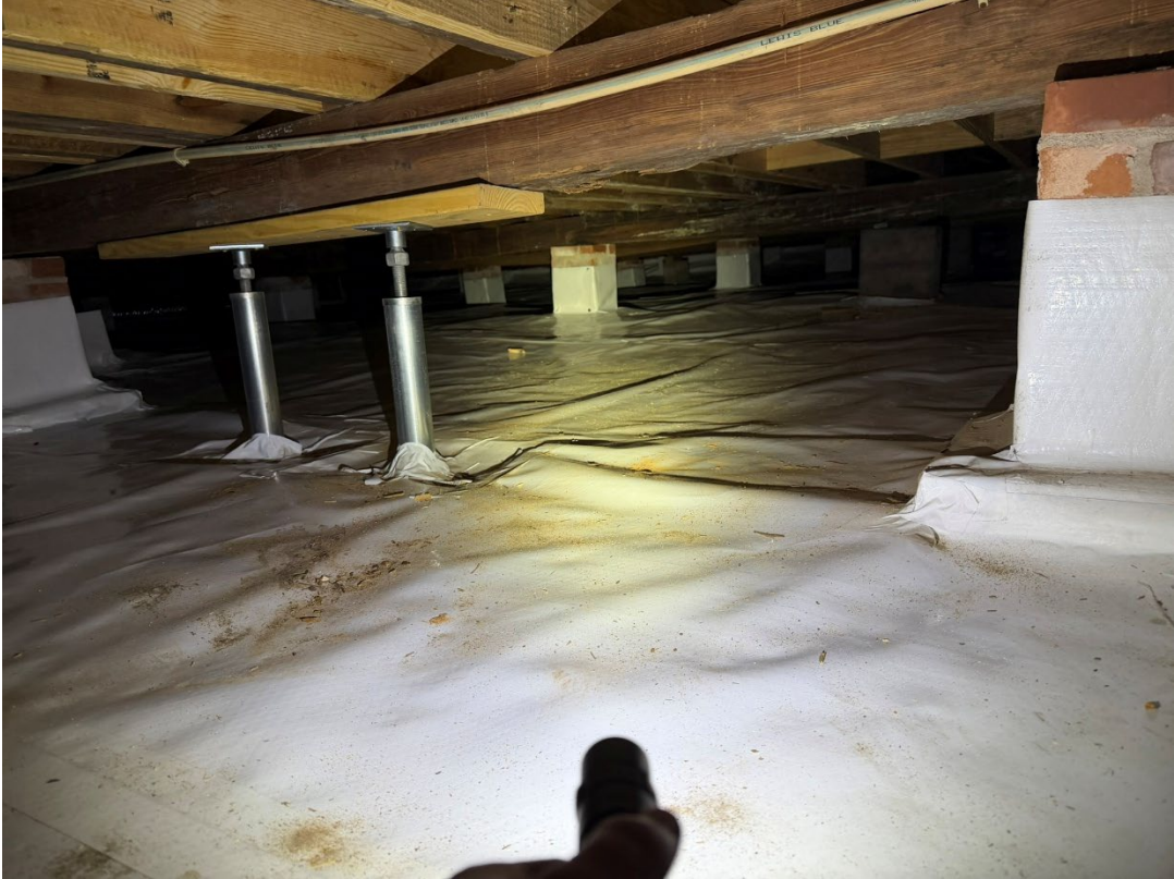
Exhibit A.2: Moisture Damaged Beams and Joists With Temporary Supports Added
