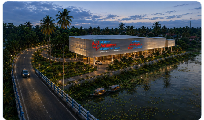
Main hospital elevation — aerial dusk view (render)
