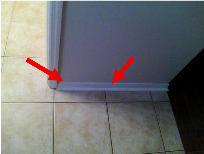
Visible hallway baseboard separation and staining adjacent to bathroom
