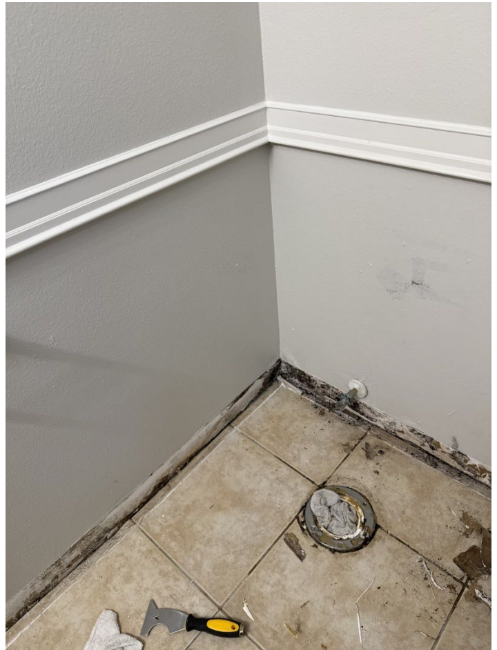
Bathroom wallboard prior to removal showed visible suspect growth near baseboard level
