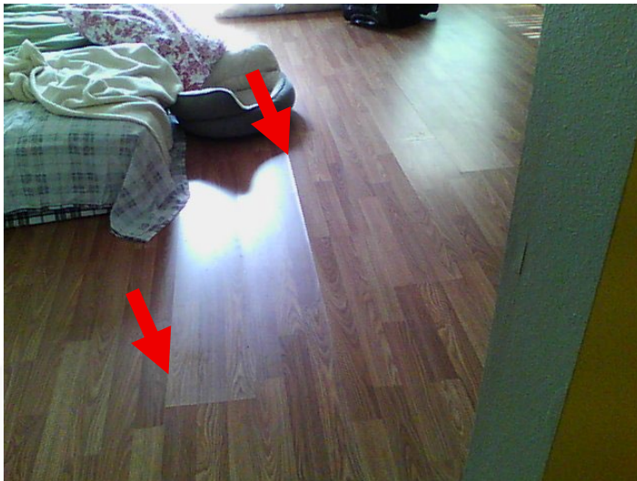
Bedroom flooring showed visible warping and crowning in multiple areas
