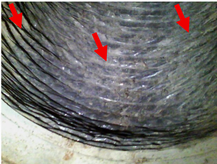
Air intake showed visible debris and suspect growth
