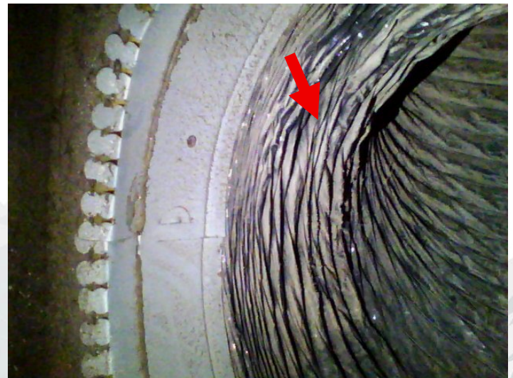
Air intake showed visible debris and suspect growth
