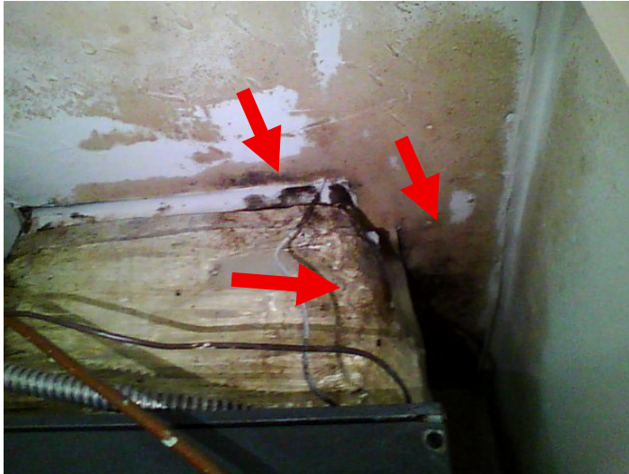
Ceiling and plenum entering the attic showed visible suspect growth
