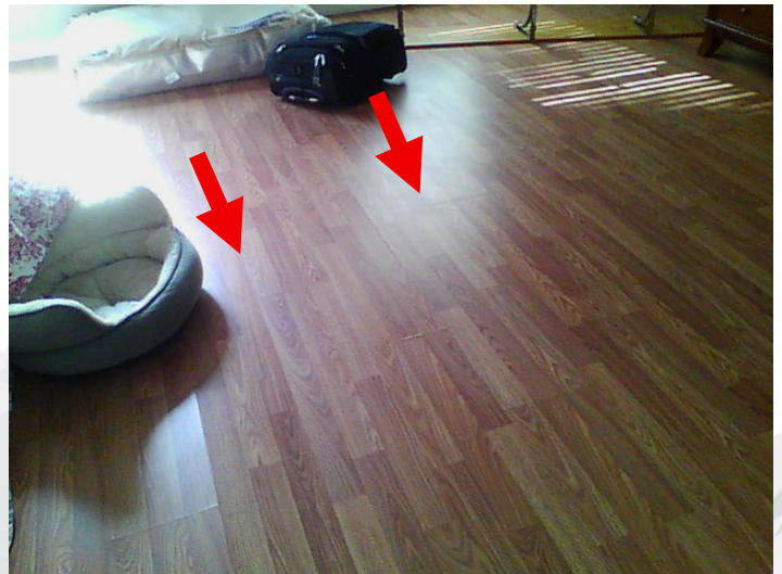
Bedroom flooring showed visible warping and crowning in multiple areas
