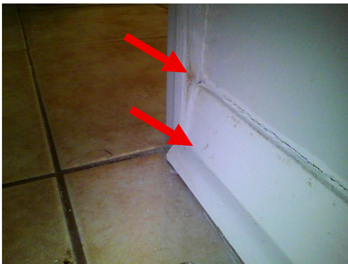
Visible Hallway Baseboard Staining
