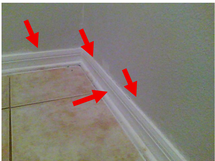
North and east baseboards showed visible separation and staining
