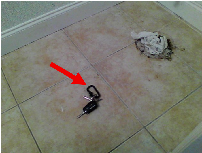
Hollow tile floor detected where keys lay
