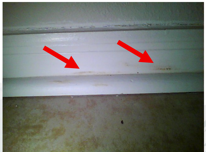
Visible Hallway Baseboard Staining
