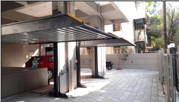
G+1 Stack Parking System, Client: Site- ANIL, Gokhale Construction, Pune
