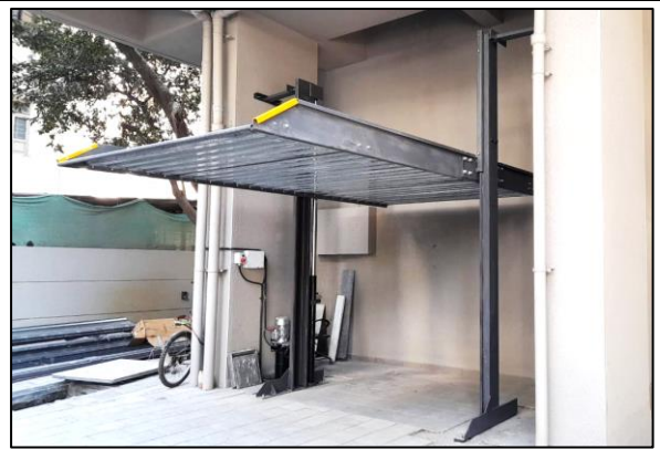
G+1 Stack Parking System, Client: Site- ANIL, Gokhale Construction, Pune
