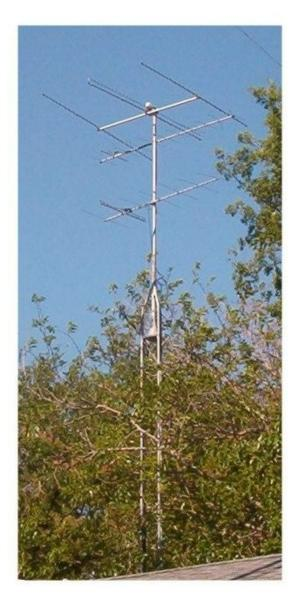
The "short tower" is 30 feet tall plus the mast. The bottom antenna is an 11-element 2-meter yagi, the middle antenna is an 11-element 222 MHz antenna, and the top antenna is a 3-element 6-meter yagi.
