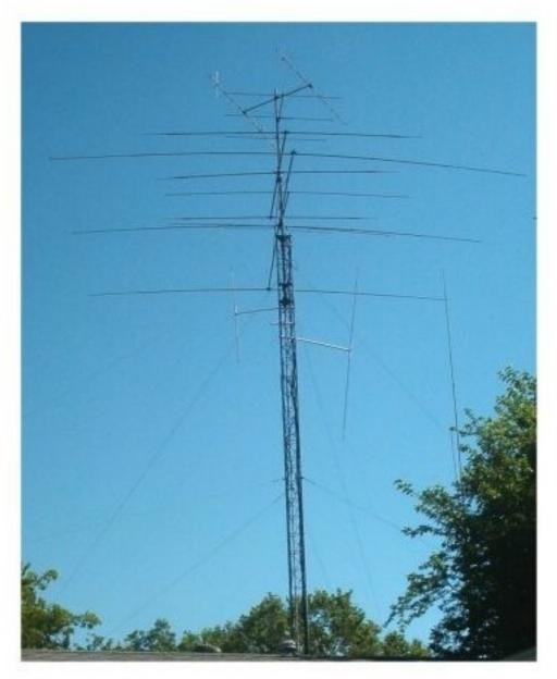
The main tower at K9STH consists of 54 feet (above ground) of Rohn 35 tower which is a tower that was specifically made for Motorola by Rohn. It is 15 inches on a side whereas Rohn 25 is 12 inches on a side and Rohn 45 is 18 inches on a side. The side-mounted antennas are (left side) 6-meter for FM operation and (right side) 10-meter for FM operation.
