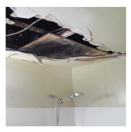
Photo of ceiling sheetrock removed. Mold is visible on the wood frame above the ceiling.
